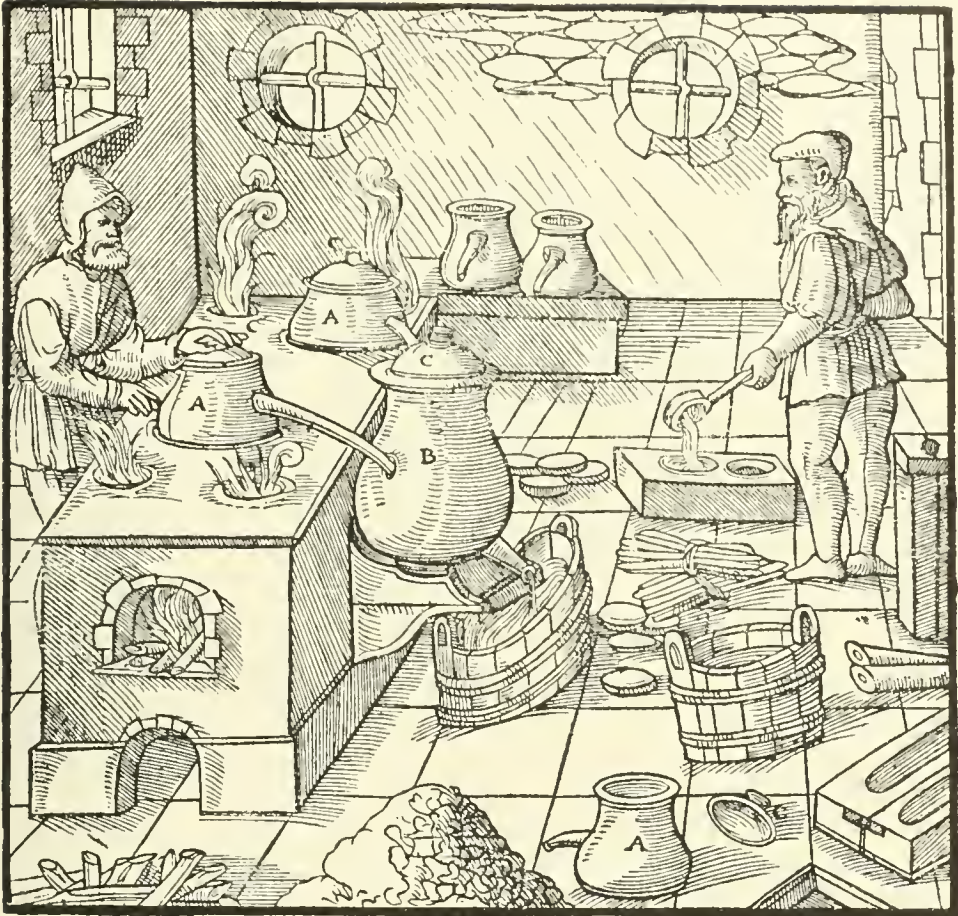
A—POTS HAVING SPOUTS. B—POTS WITHOUT SPOUTS. C—LIDS.
